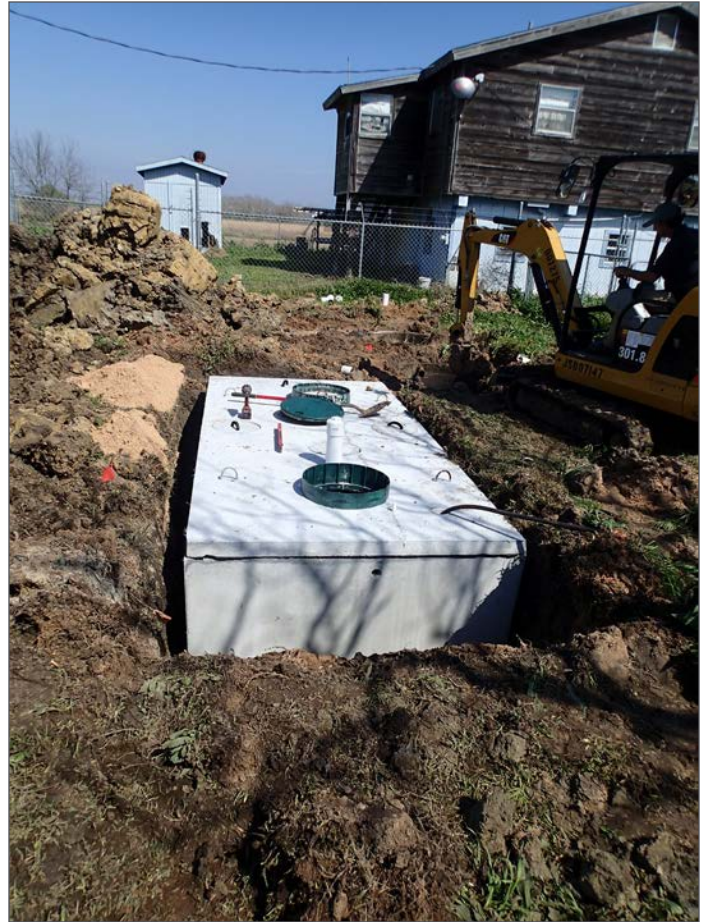
Failing OSSF system replacement installation. Photo by Ryan Gerlich.
